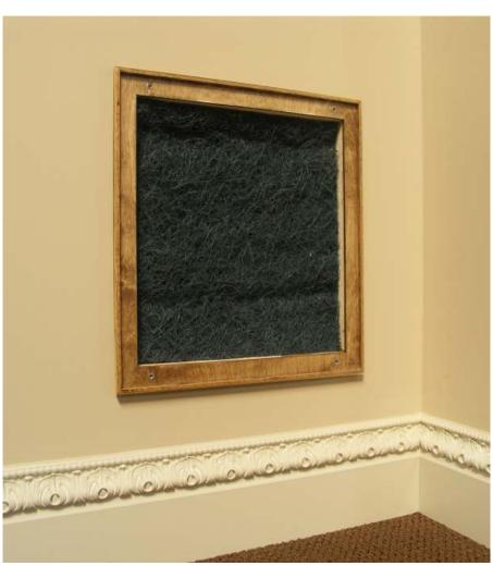
Attach the grille cover with the included brass thumb screws.
